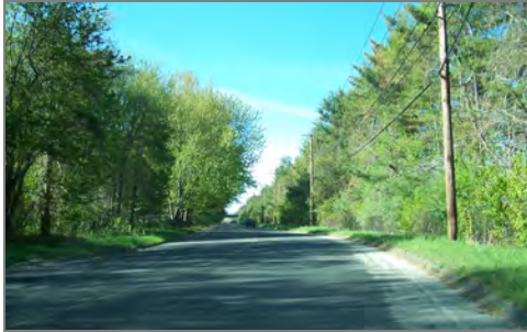
The gateway to the Merritt Corporate Park does not convey the image of a modern, corporate park. Improvements are planned. The road is wide enough to provide bicycle lanes.
