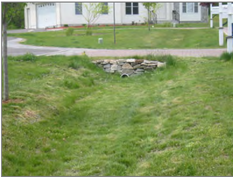
Vegetated swales that promote infiltration.
